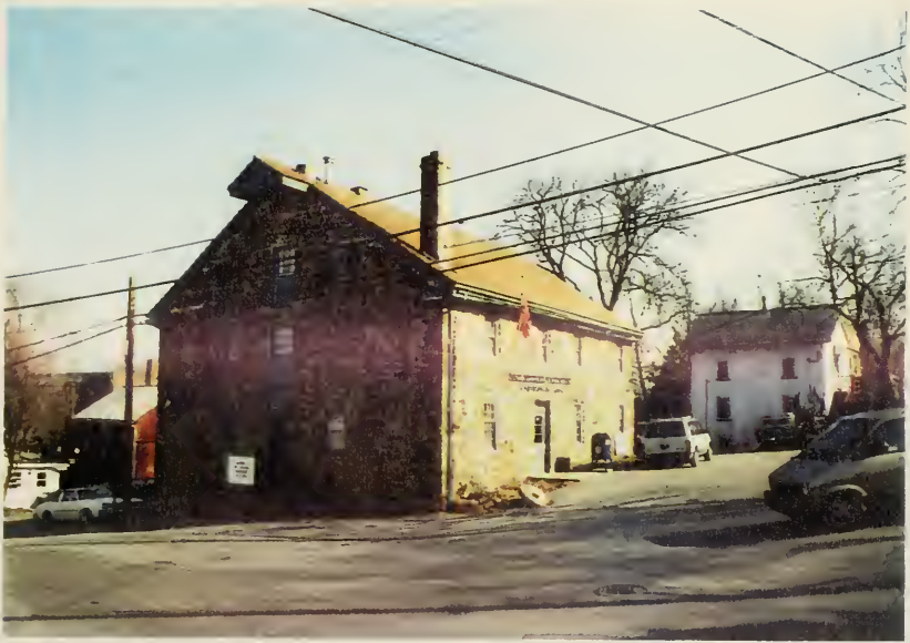
Fig. 115 Crisman's Mill at the intersection of Hares' Hill Road and Kimberton Road. • The mill now serves as the township's post office. Photograph by the author, 1995.
